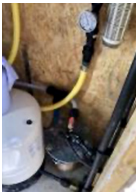
Head of the borehole and flow through expansion vessel
