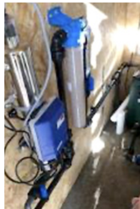
Photograph of the UV and Fine Filter after the tank
